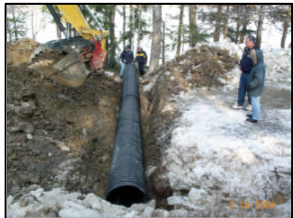
Sheldon Beal, Dave Brooks, Bob Beal and Edith Brooks observed the placement of the culvert in the trench near the Ellis camp.
